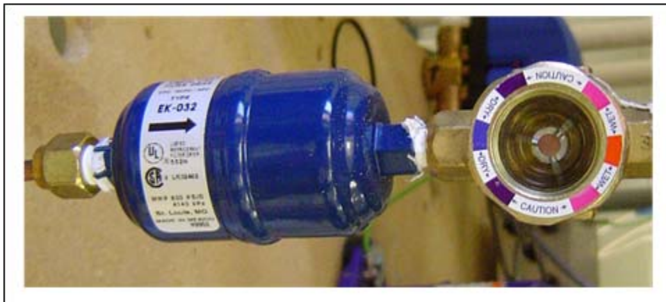
Figure 2.10: Filter drier with sight glass
