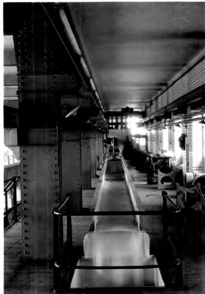
EXPERIMENTAL STEEL FLUME, LOOKING U.S. FROM THE BOTTOM END.
