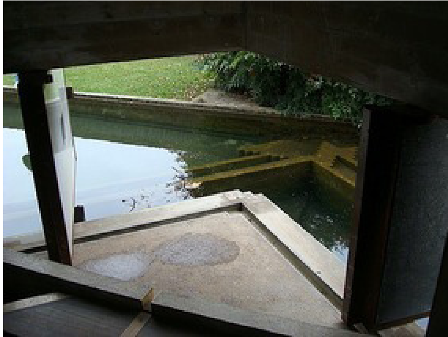
Figure 8: The chapel is open to water and the memories below.
