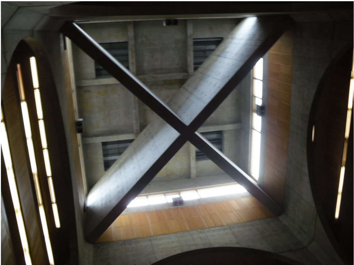
Figure 11: Central void with concrete trusses.
