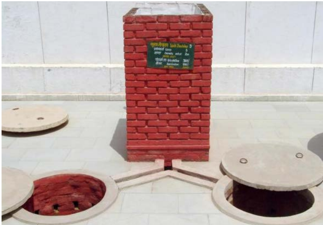
Figure 1: Sulabh's Two-Pit System [1]
