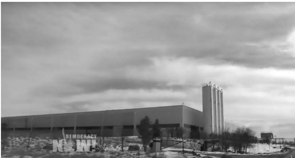
Figure 2.4 Exterior view of the Nestlé Waters Ice Mountain bottling plant near Stanwood, Michigan.
