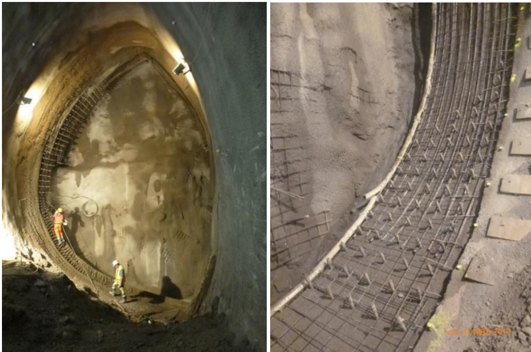
Figure 5: Construction shear dowels
