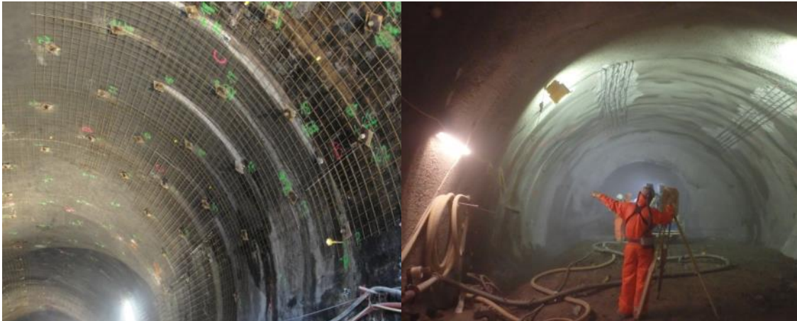
Figure 2: Subsequently added strengthening of the shotcrete layer
