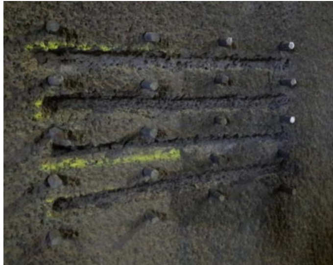
Figure 4: Indented construction joint - performed
