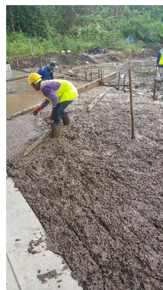
Figure 3 – Overlay in truck yard
