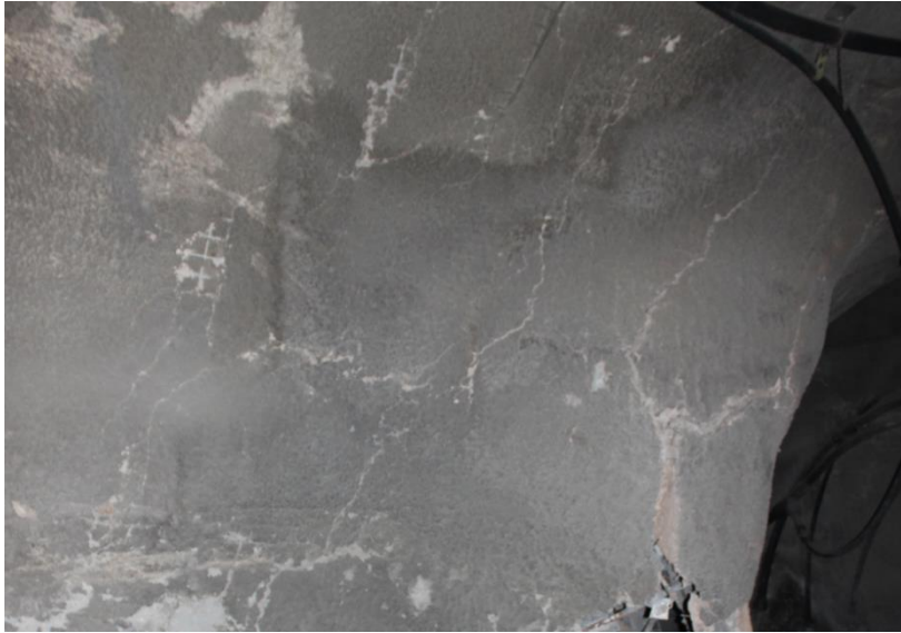
Figure 15 – Mesh reinforced shotcrete response to sudden low energy demand. Fracture intersections correspond to the location of reinforcement elements.
