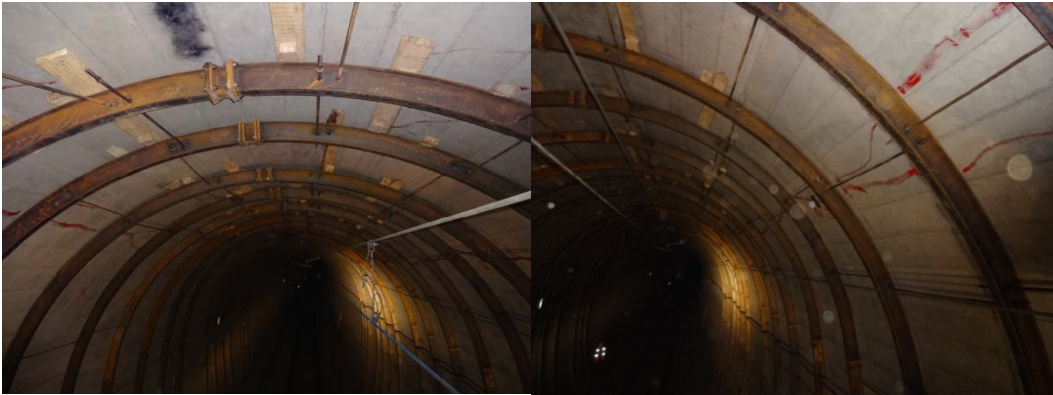
Figure 11 Temporary steel-rib arch for supporting vert severe damaged lining section
