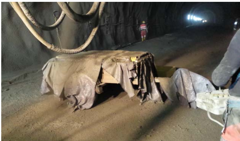
Figure 3. Shotcrete panel production on site
