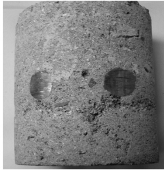
Dry-mix shotcrete, #4 bar, sand lenses.
