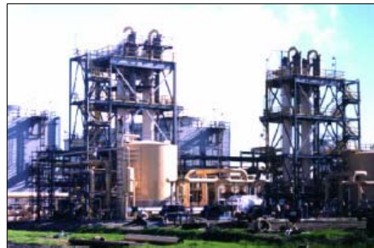
Figure 3: 4,600 m 2 self-cleaning heat exchanger surface replacing 24,000 m 2 conventional surface.
