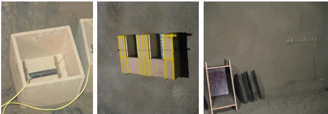
Fig. 4: a) Test box equipped with SSM-1 for shrinkage test, b) Formwork installation, c) Steel formwork with sprayed-in formwork
