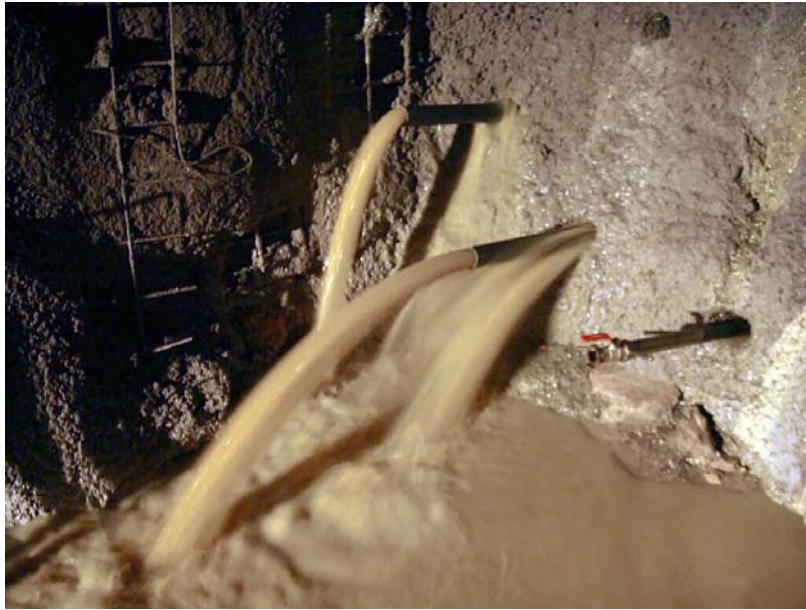
Fig. 10: Water flow out of the working face supported with sprayed concrete
