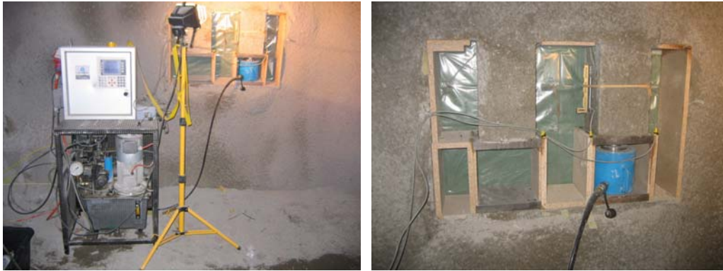
Fig. 5: a) Mobile compression test equipment, b) specimen with loading (hydraulic cylinder) and measuring device (LVDT) in the tunnel side wall
