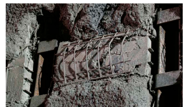
hiDCon element in yielding tunnel support system, 15% deformation
