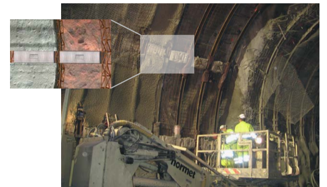
St. Martin la Porte access tunnel: Detail of hiDCon elements within the yielding tunnel support
