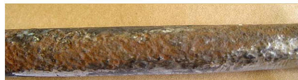
Fig. 1-b) External Tube Corrosion
