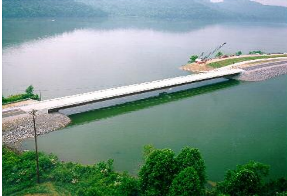
Figure 1. State Route 53 over Martin Creek
