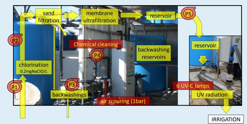
**<u>REAGENTS</u>**: for chlorination, for chemical cleaning (fresh water, NaClO, NaOH)
