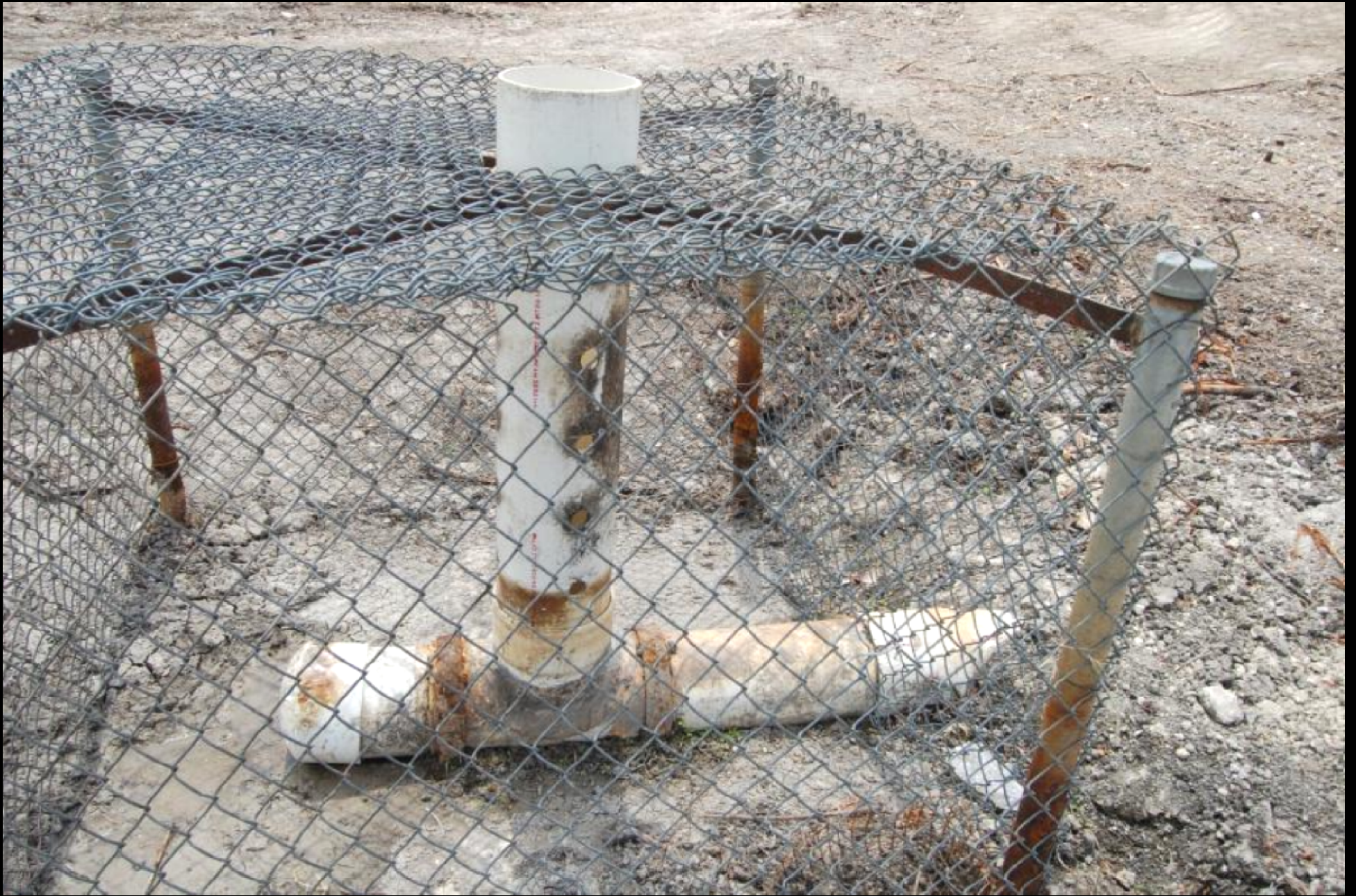
Existing Pond Outlet Control Structure – Austin, TX
