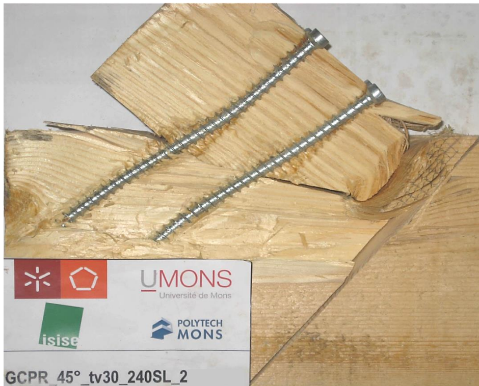
Fig. 9 Double plastic hinges of FTS implemented in the rafter at the bottom-notch surface.
