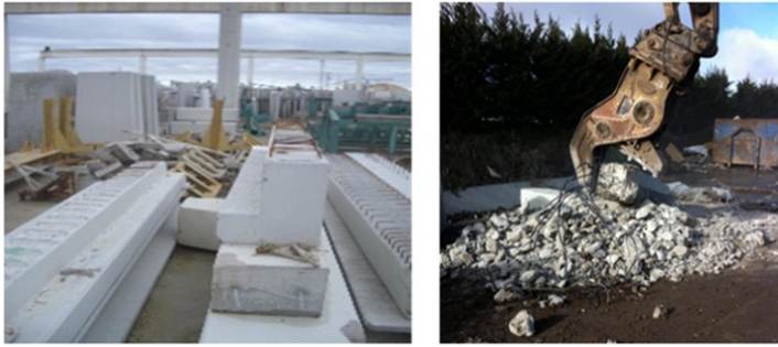
Fig. 2 Waste landfill site for precast reinforced concrete and their crushing process.
