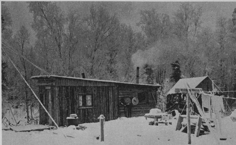
A homesteader's cabin southwest of Wasilla. This family lived in the tent on the right during their first winter. During the second winter they lived in the small cabin of horizontal log construction which now forms the back room of their present home. Land clearing is their ever-present worry.
