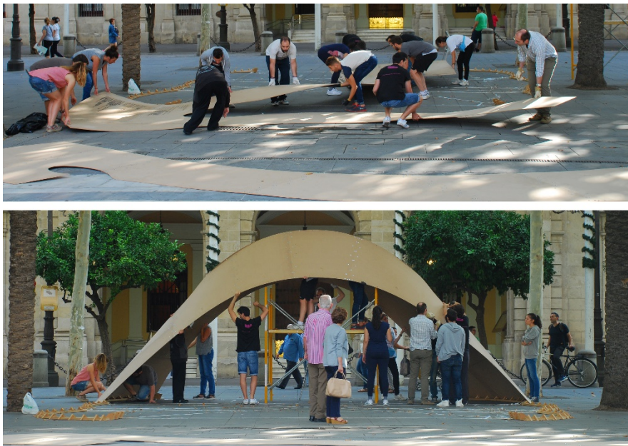
Fig. 3. Different stages of assembly of Fablab SSFS Pavilion Plaza Nueva in Seville
