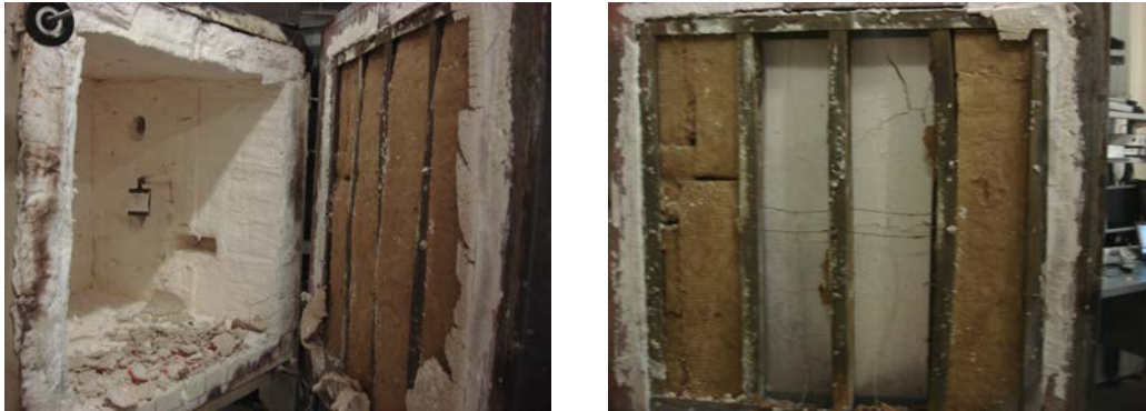
(a) Exposed side after the end of the test. (b) Exposed side after the end of the test.
