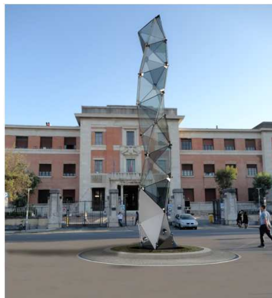
Fig. 2: Example of 15.00 meters tall HYGLASS installed at a roundabout in front of the School of Engineering main building (Pisa), taken from Froli and Laccone (2018)
