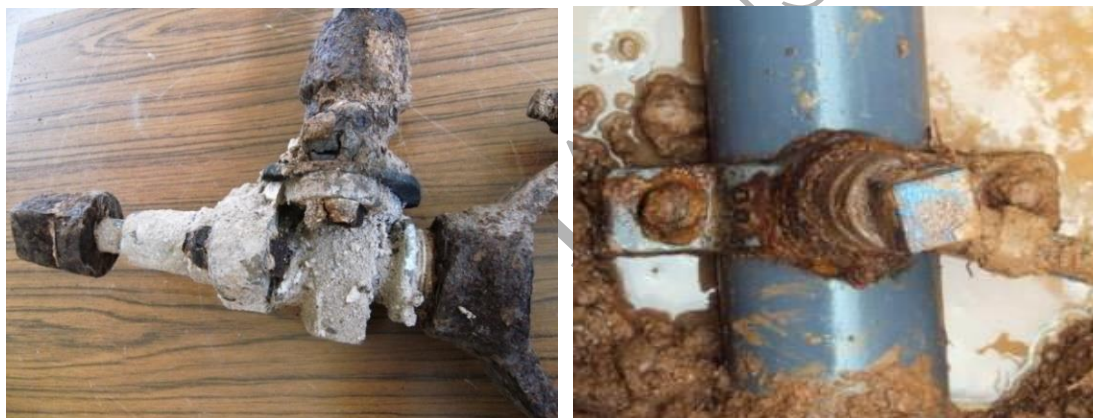
Fig.1. Plumbing system examined
