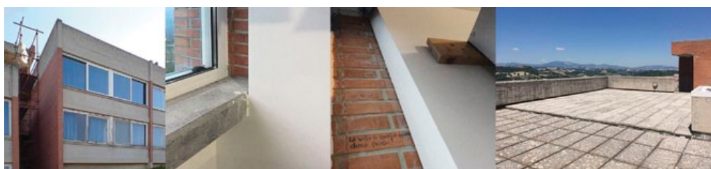
Figure 8. After the pilot site, from left to right: new window, “cold wall” insulation, slab cover.
