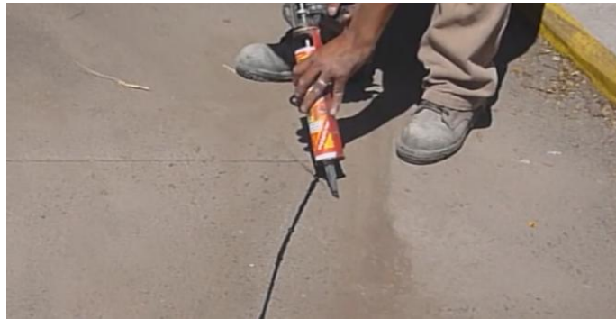
Picture 15. Applying sealer
