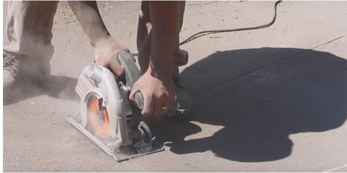
Picture 14. Cutting a slot
