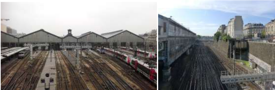
Figure 5 and 6: Depressed railways and the perspective they create. Sources: the authors (Fig.1), Mbzt © (Fig.2).
