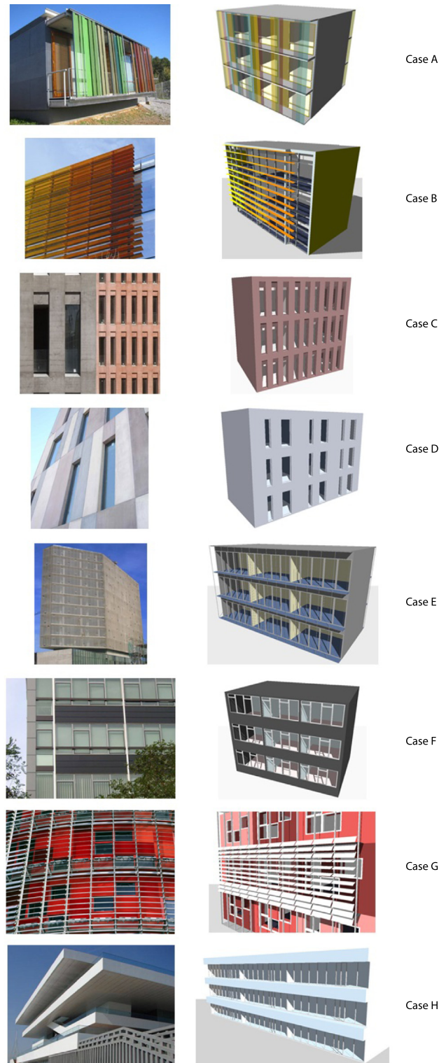
Fig. 1. Facades of the studied buildings. Real pictures and thermal models.
