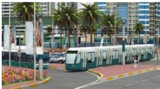
Figure 2 An LRT System running on-street.
