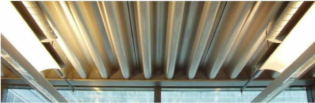
Figure 1. Profiled stainless steel decking [12].
