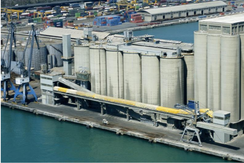
Figure 12. Portcemen terminal in Port of Barcelona. It can be seen the 12 silos, the conveyor belt and the loading and unloading equipment of the terminal. Source: Google Maps
