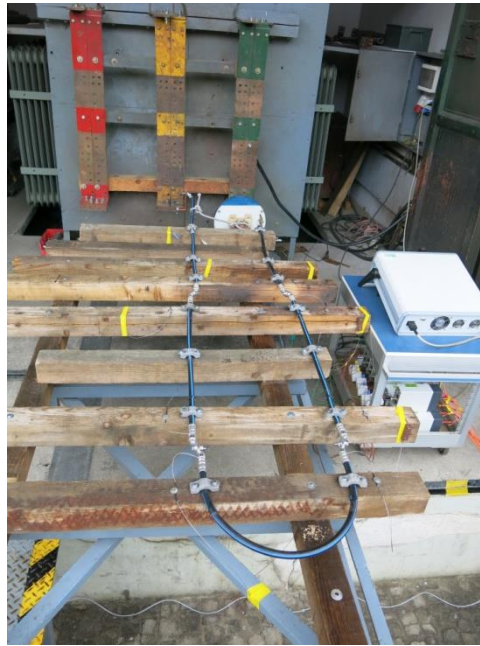
Figure 2.4: Short-circuit test assembly for low voltage connectors
