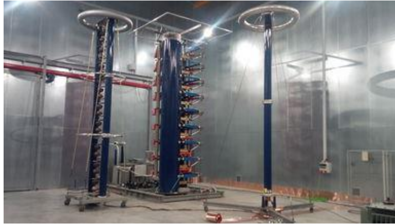
Figure 1.6: Screened high-voltage laboratory [15]
