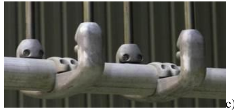
Figure 3.12: The five models of substation connectors analysed in this section. a) T-type connector J285TLS, FS and RS with a scale factor 1:1.745. b) T-type connector S285TLS, FS and RS with a scale factor 1:1.745. c) Coupler connector J40S33PK. d) Double coupler connector J40S33DPK. e) Duplex T-type connector Z12T390D9DLSP.
