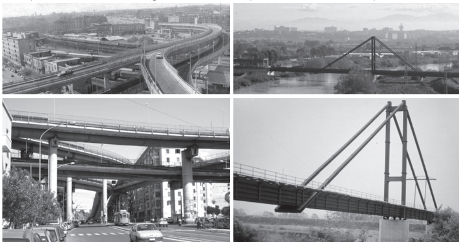
p.7 - Comparison 5 left: San Lorenzo Viaduct and the abundance of giant steel devices (F. De Miranda, CMF, 1972) right: one of Magliana service and pedestrian Bridge and the Tiber crossing with a few architectural signs (Cimolai, 1975)
