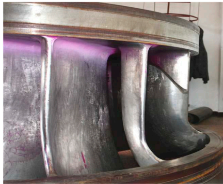
Figure 1. Francis turbine blade failure case reported by D Frunzäverde, 2010 [7].
