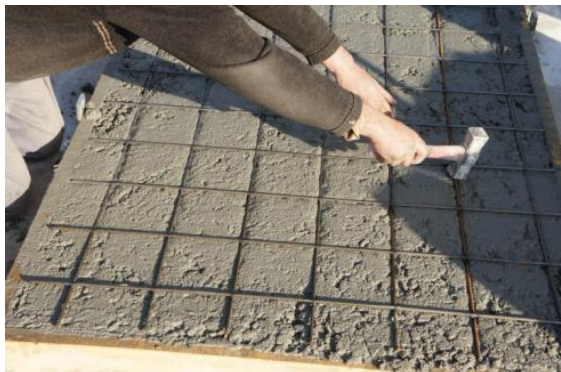
b) Detail of the crack inducer (short span)
