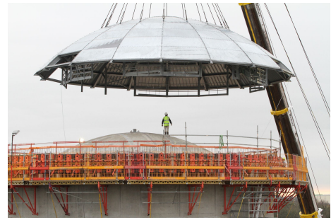
(a) View during construction (March 2015) (b) External dome lifting (November 2015)
