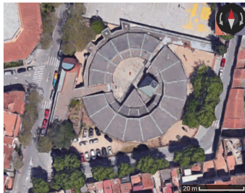
Figure 3.1: Pilot installation image
