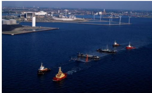
Figure 5: Fehrmanbelt, transport of the tunnel elements - Font: https://femern.com/en [37]
