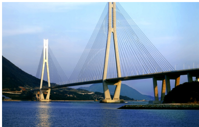
Figure 16: Cable Stayed Bridge – Font: http://global.kawada.jp/bridges/cablestayed.html
