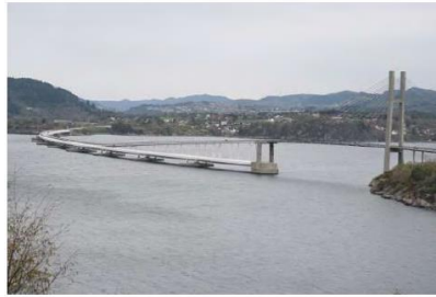
Figure 17 – The Nordhordland floating Bridge - Font: The Nordhordland Bridge – Twenty years in service ; [76]: pp 330-339
