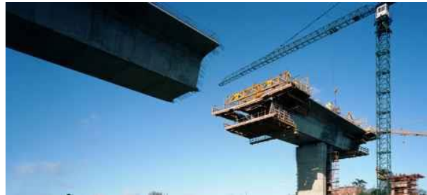
Figure 13 – Balance Cantilever construction method - Font: http://www.bridgesofdublin.ie/bridge-building/types/cantilever/ ; [33]
