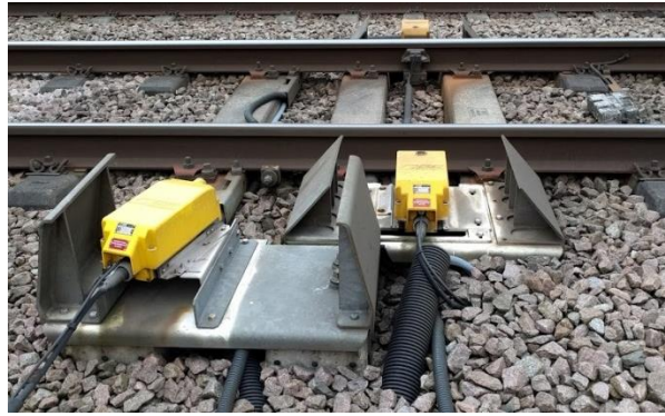
Figure 9: HABD on a UK high-speed line
