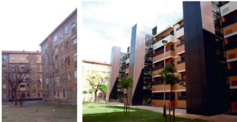
Fig 4. Public green zone and towers of installations
