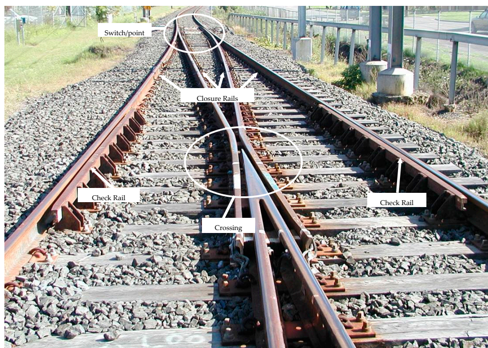
Figure 1. Typical turnout geometry.
