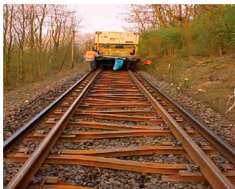
Figure 3. Y-Steel-Sleeper.
