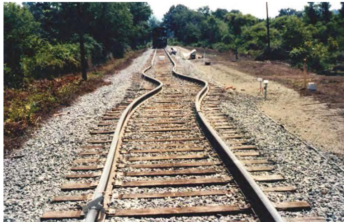
Figure 1. Rail buckling due to lateral movements of sleepers, commonly found in timber and steel sleepered tracks (Kumaran, Devdasand Krishnan 2003)
