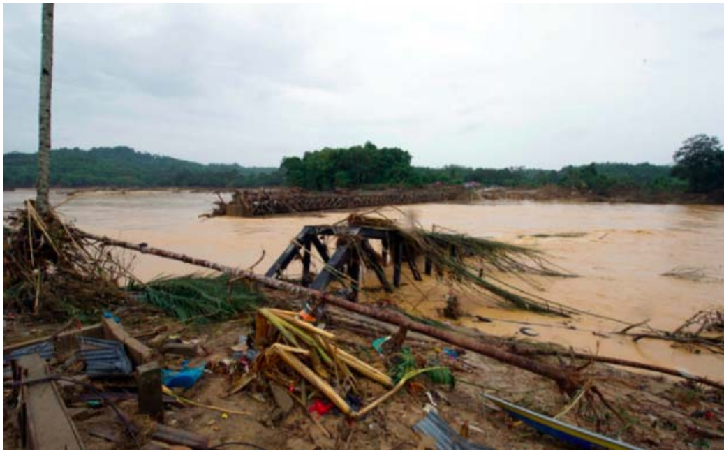
Figure 5. Malaysia East Coast Line railway bridge which crosses Nenggiri River in Kemubu, Kelantan was completely lost due to massive flooding in December 2014 (courtesy: Malaysia Department of Public Works).
