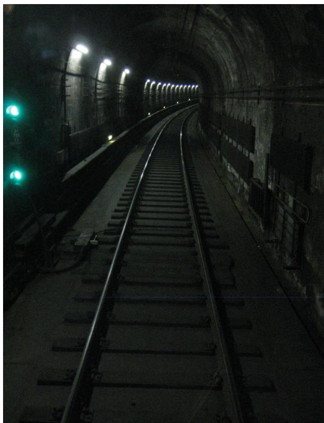
Fig. 2 A typical curved track where a high-pitch corrugation on low rail tends to occur
