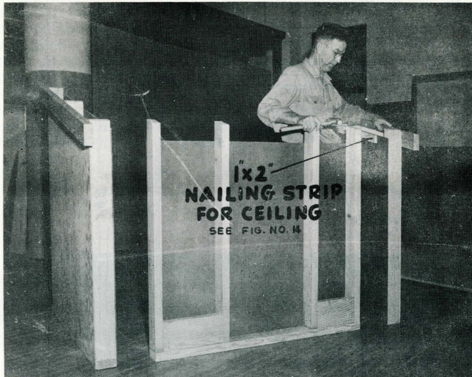
Figure No. 11 Rear wall being assembled to sides. Note that plywood on rear wall has not been nailed in place.
