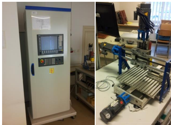
Figure 3. Control cabinet and three-axes milling machine [4]
