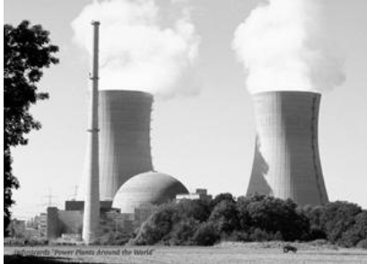
Nuclear power station
