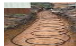
Ground source heat pump
