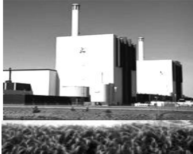
Biomass plant & Energy crop
