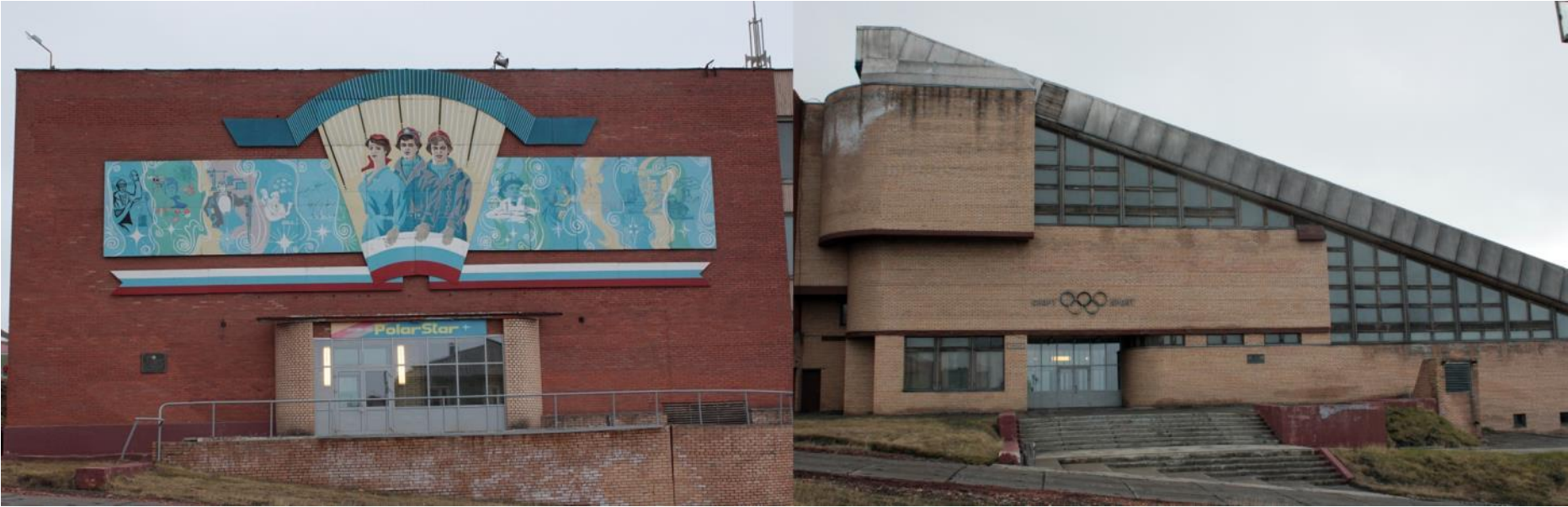
Figure 18: Barentsburg Sports and Cultural Centre (montage), June 2013
