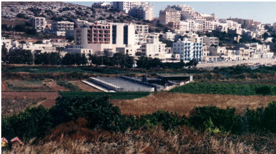
Photo 3.1: Concrete tanks of land-based Fish farm next to nature reserve.
